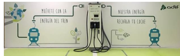
Electric recharging points powered by regenerative brake energy
